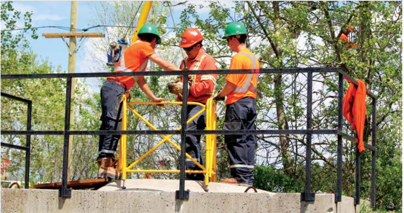
Two apprentice power line maintainers going through a confined space entry/rescue exercise with a journeyman line maintainer, during a North American Occupational Safety and Health Week/Tool and Equipment Inspection Week event. Photo courtesy of Hydro Ottawa.
