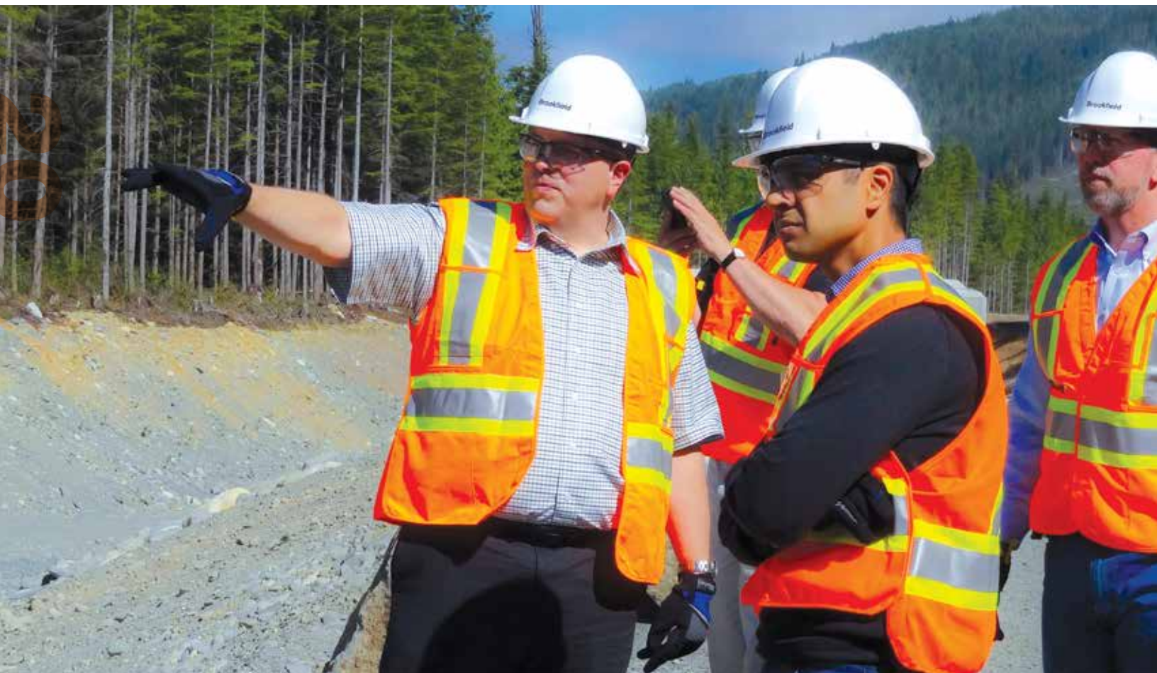
Caption: Brookfield employees talk about safety on site. Photo courtesy of Brookfield Renewable Energy Group.
