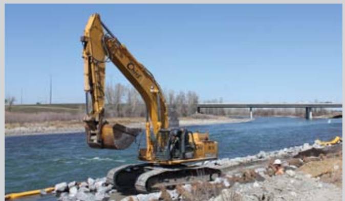
ENMAX Power completed a riverbank stabilization project along the banks of Calgary's Bow River in 2010, creating a permanent structure of rock and vegetation to protect power transmission and distribution from future erosion, while creating an attractive natural habitat for wildlife.
