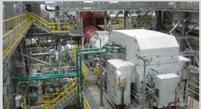
The new steam turbine generator, and other auxiliary systems, at the Fort Nelson Generating Station.
