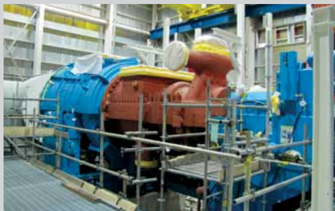
Steam turbine and the generator at the biomass cogeneration unit at NewPage Port Hawkesbury (NPPH) mill.
