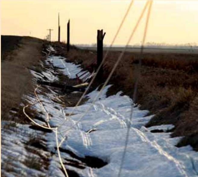
A spring storm in southern Alberta causes significant damage to a FortisAlberta power line.
