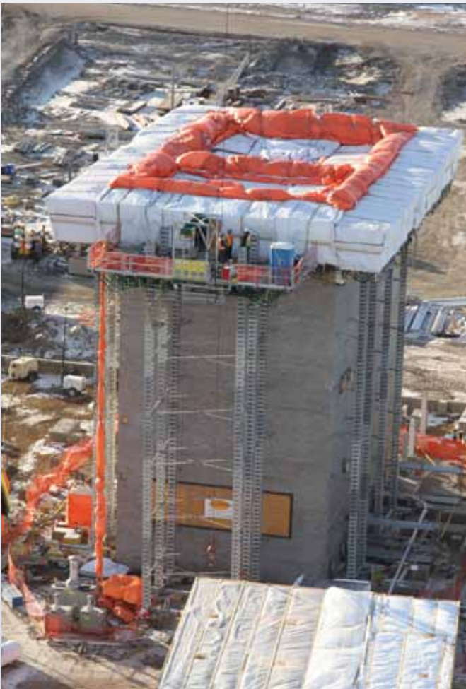
CO 2 and SO 2 Absorber Construction at the Boundary Dam Integrated Carbon Capture and Storage Demonstration Project.
