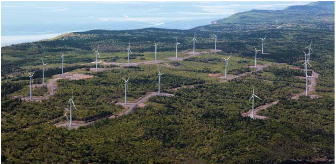
Completed in 2010, the Digby Neck Wind Farm supplies up to 10,000 homes. Photo courtesy of Nova Scotia Power Inc.
