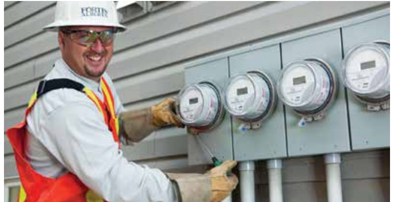
Toronto Power line technician Pete Patton installs an automated meter. Photo courtesy of FortisAlberta Inc.
