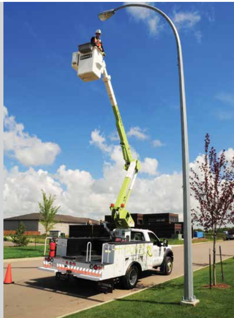
Worker makes repairs in residential community. Photo courtesy of FortisAlberta Inc.
