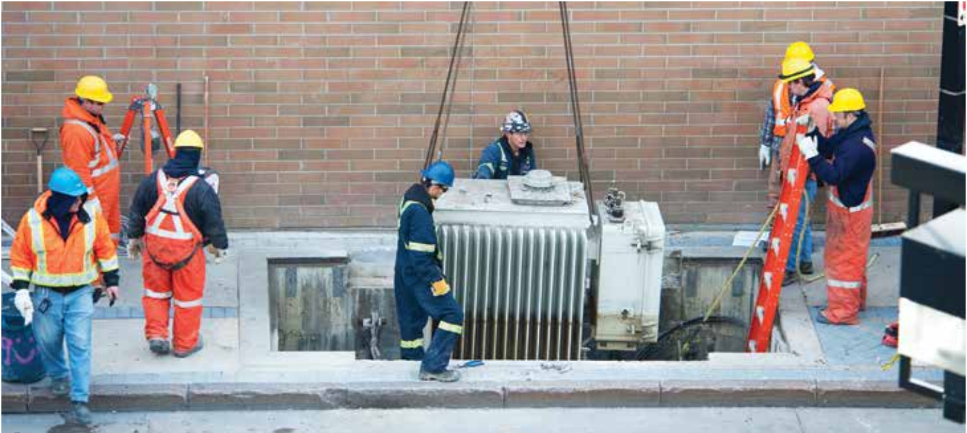
Manitoba Hydro crews install new equipment in a vault beneath Graham Avenue in downtown Winnipeg as part of the utility's infrastructure renewal efforts. Photo courtesy of Manitoba Hydro.
