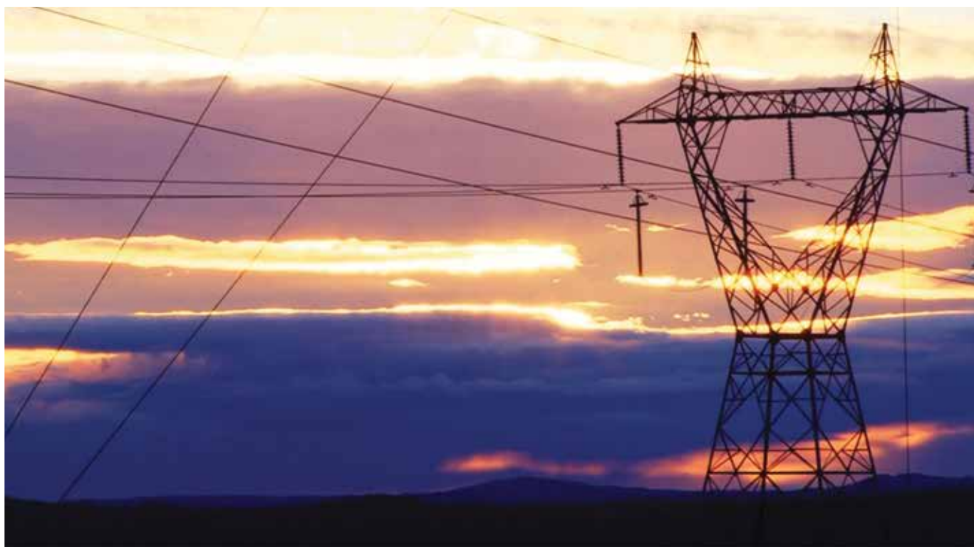
Transmission Lines and the skyline. Photo courtesy of Nalcor Energy.
