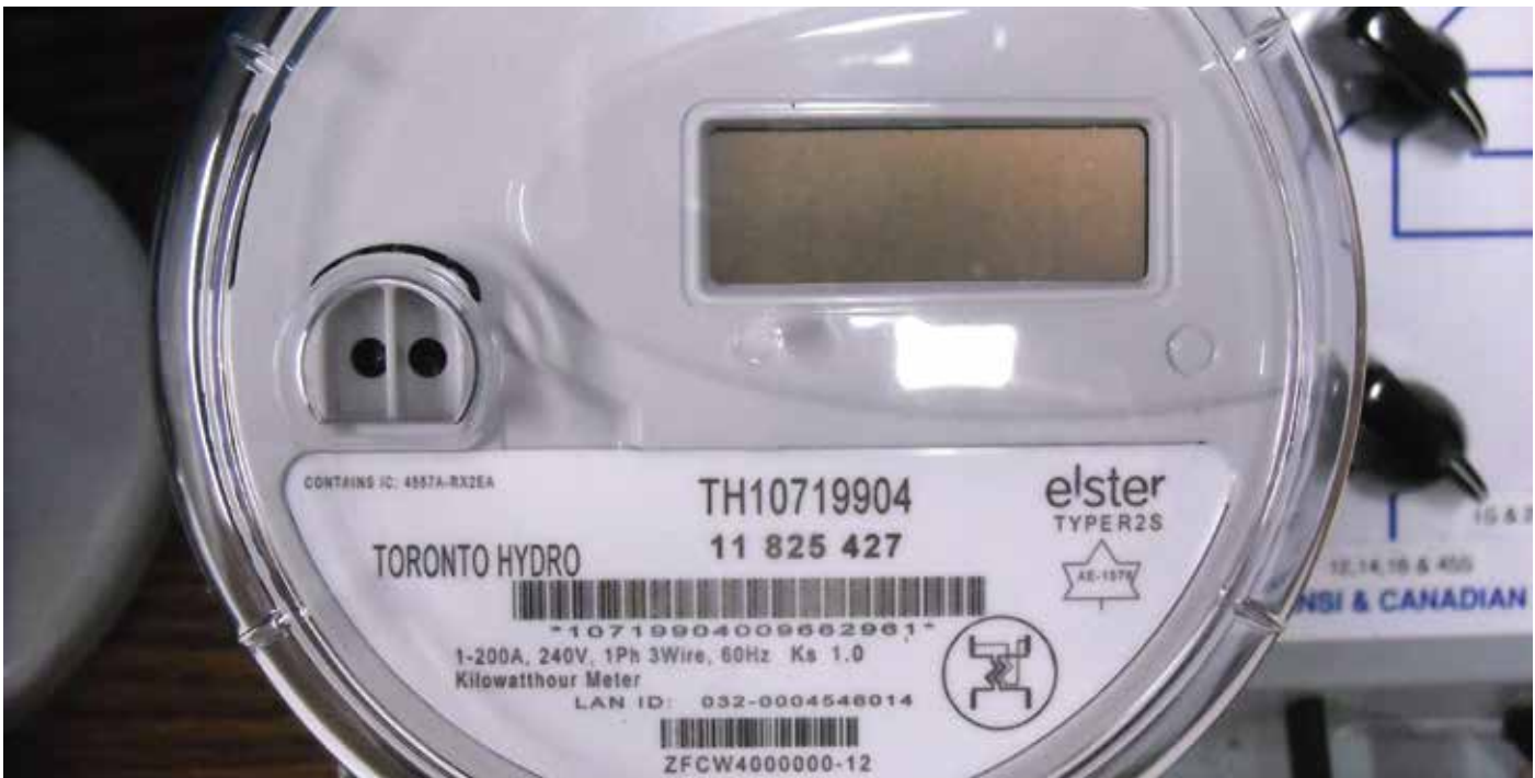
Toronto Hydro Corporation has converted 99.7 per cent of its meter population to Smart or Interval Meters. Photo courtesy of Toronto Hydro Corporation.
