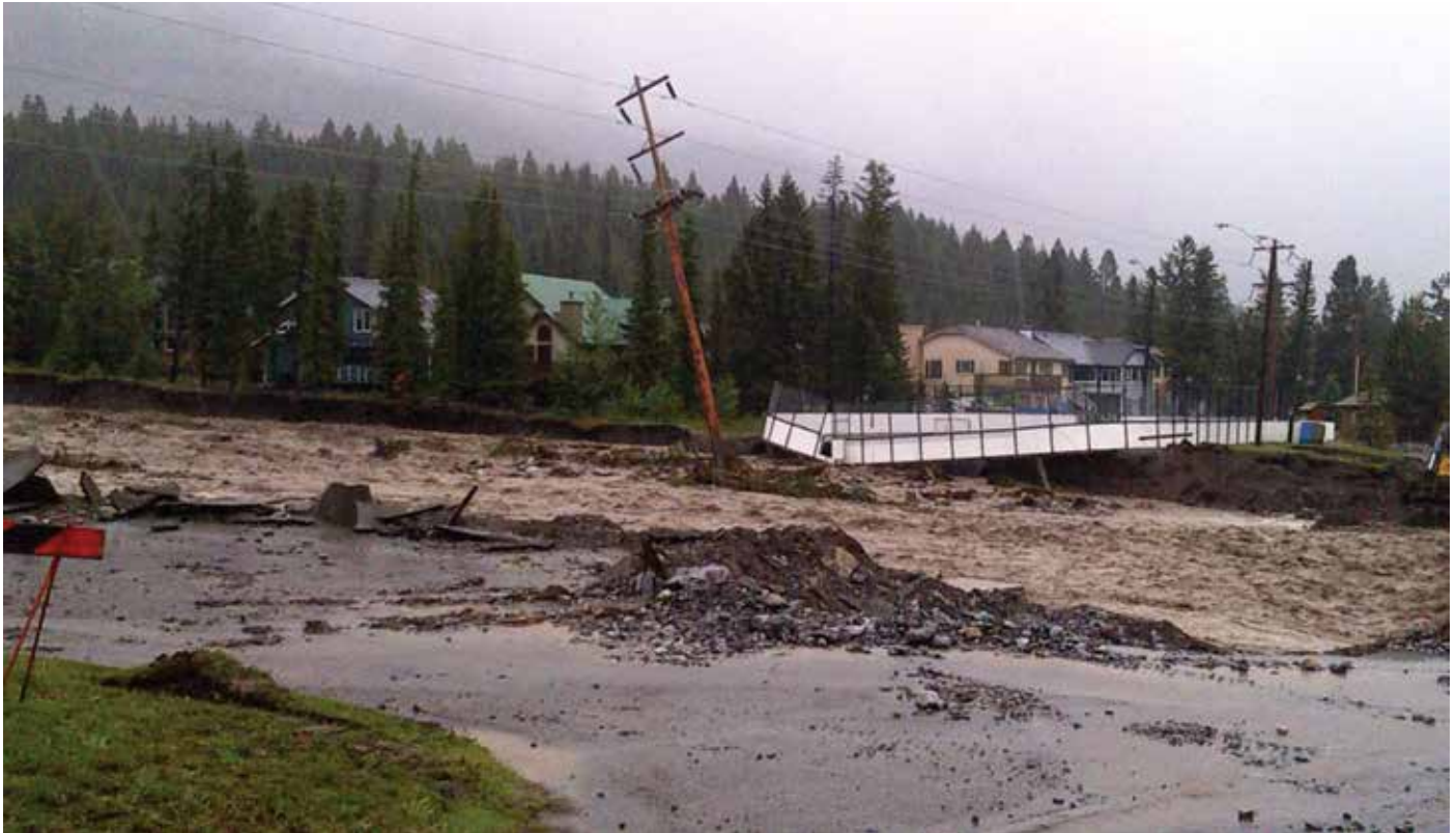
An AltaLink transmission line in Canmore, Alberta during the 2013 flood. Photo courtesy of AltaLink.
