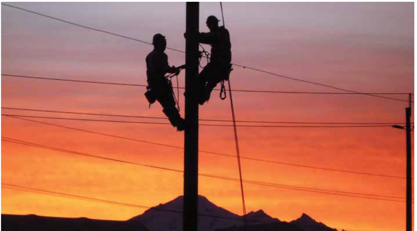
BC Hydro power line technicians work to ensure power. Photo courtesy of BC Hydro and Power Authority.
