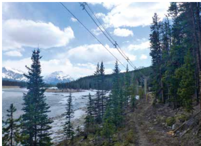
A section of the newly-installed aerial spacer cable system along the Astoria River. Photo courtesy of ATCO Electric.
