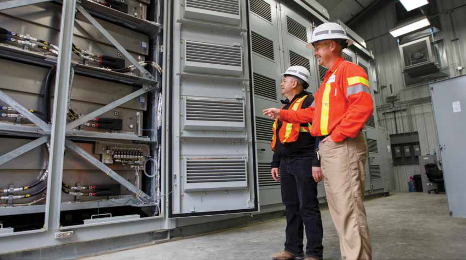
Trevor Wareham, BC Hydro Electrician Sub-foreman, and Vlad Kositsky, BC Hydro Project Manager, inspect one of four banks of sodium-sulphur battery modules. These four banks of battery modules, linked together, create the one megawatt capacity. Photo courtesy of BC Hydro and Power Authority.
