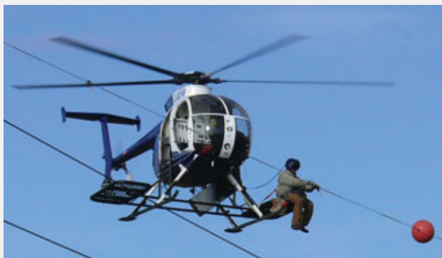
AltaLink's north field crew installs bird markers along a portion of its transmission line that runs through Lois Hole Provincial Park in Central Alberta.
